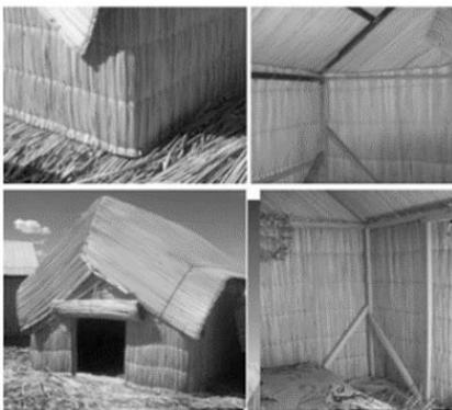
Fig. 1. Uros’s totora house details. Adapted from [6].
