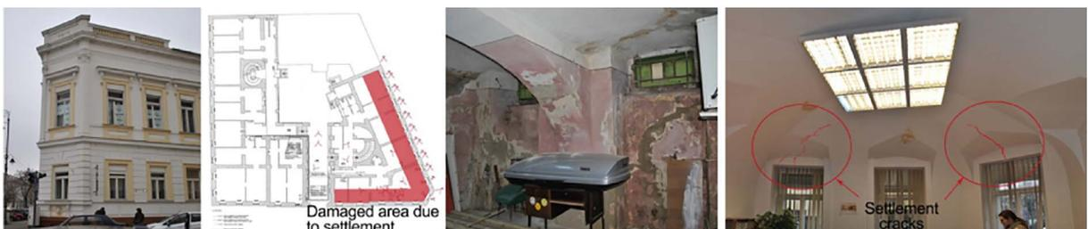
Fig. 2. Severe damages by heavy rain and terrain settlement at a heritage building in Arad, Romania.
