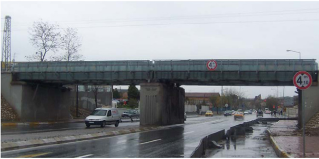
Fig. 1. A general view of the bridge.
