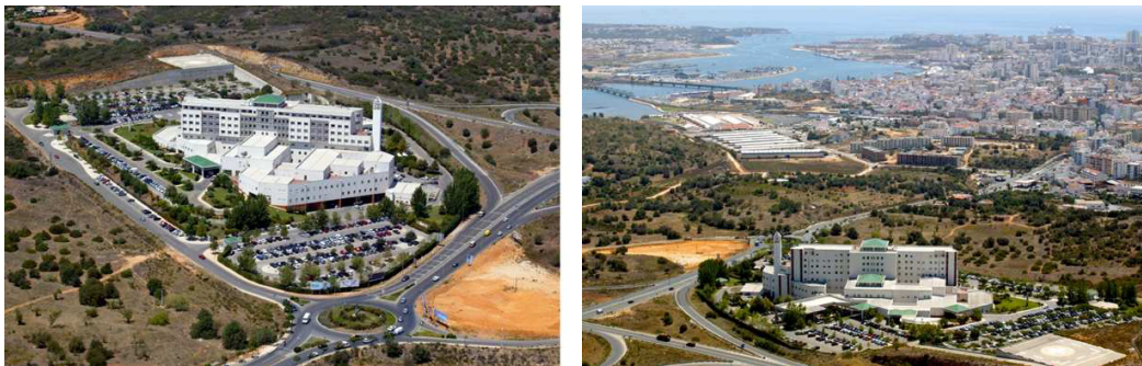
Fig. 1(a) Location of the Hospital; (b) Regional insertion of the Hospital
