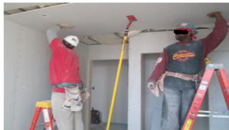
Fig. 1. Use of the tool at a construction site.
