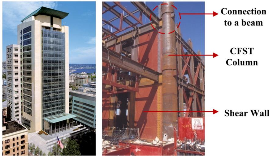
Fig. 1. Example of application of CFST member to a building column (U.S. Federal Courthouse, Seattle, WA, USA [1]).
