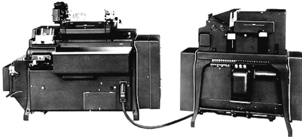
Fig. 1. Early office machines—tabulator (left) and reproducing gang punch (right).
