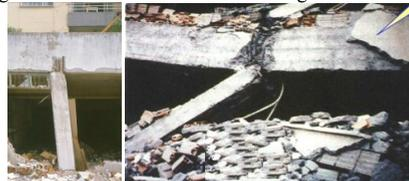
In picture 2 short columns with window openings and landings beam formed inadequacy of the stirrups in the column caused brittle fracture.
