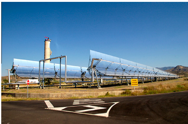
Fig. 1. General view of the DISS test facility, a parabolic-trough solar thermal power plant owned by Plataforma Solar de Almería (CIEMAT).
