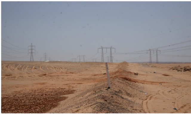
Fig. 1. Fayoum gas pipeline geometry, where the three transmission lines are parallel or crossing it.
