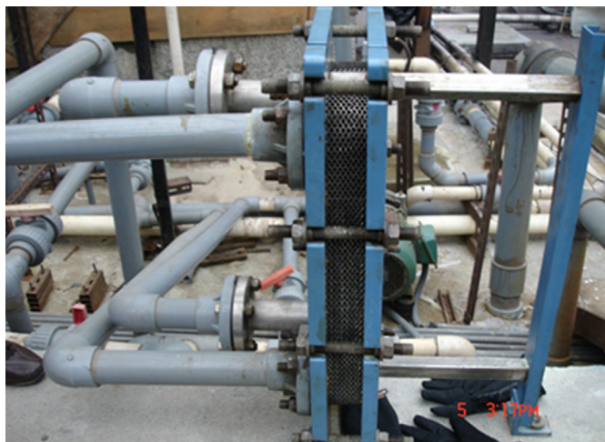
Fig. 2. Geothermal drainage by drilling to the rock mass 1000 m underground and the plate heat exchange system.
