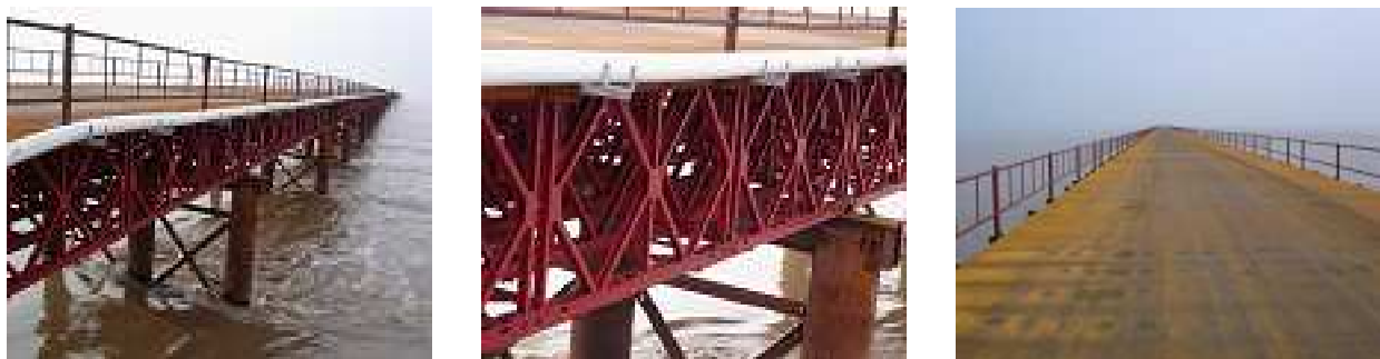
Figure 1. Temporary bridge for constructing Hangzhou bay bridge
