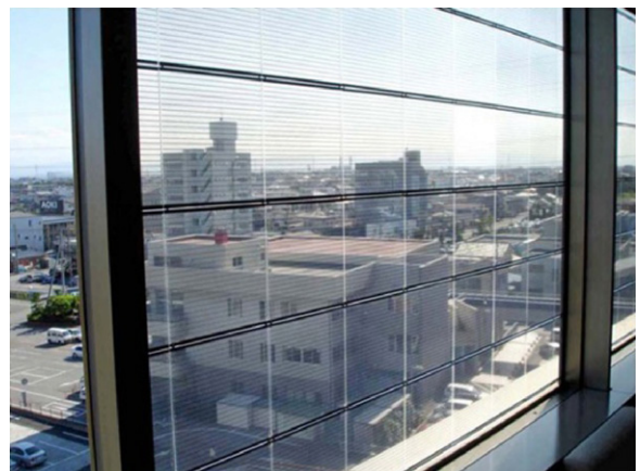
Fig. 3. Effect of amorphous silicon thin-film photovoltaic modules.
