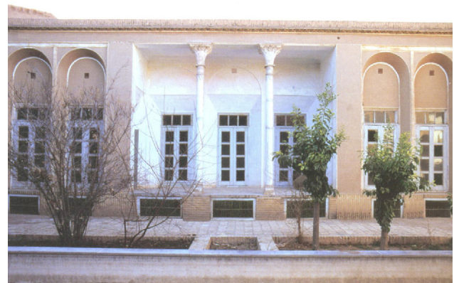
Fig. 3. An eyvan in Yazd. Source: Haji-Ghasemi (2004).
