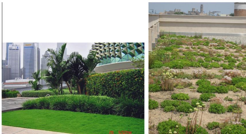
Fig. 1. Left: Intensive green roof, Singapore 2007. Right: Extensive green roof, Lleida 2010.
