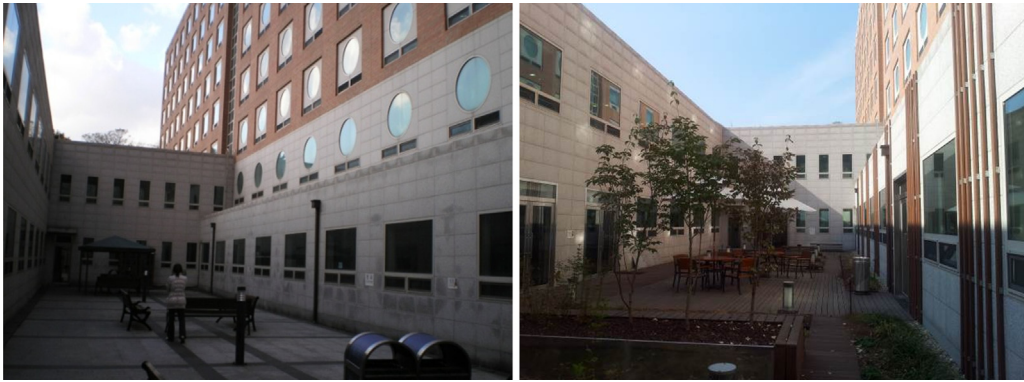
Fig. 1. Site conditions before (left) and after (right) the refurbishment using vegetation, wood decking and street furniture.
