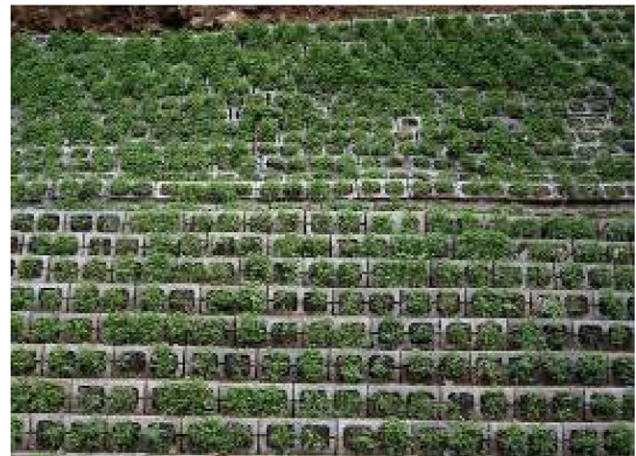
Fig. 1. Illustrations of the conventional technique (top) and air brick planting technique with a stairstep pattern (middle) and a smooth slope (bottom).
