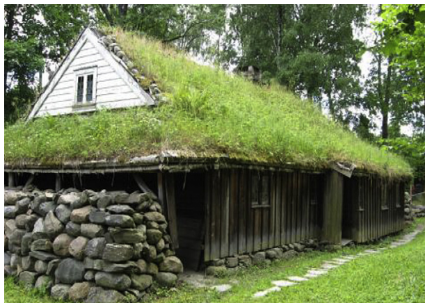
Fig. 1. Traditional green roof with native vegetation in Norway [1].
