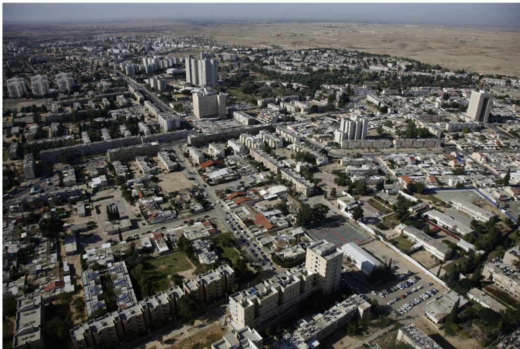
Fig. 2. An aerial photo of Beersheba's inner neighborhoods composed of low-density buildings, with the newer neighborhoods at the outskirts. Source: with permission from Lowshot.co.il.
