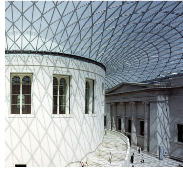
Fig. 2. Triangle meshes in freeform architecture. Laying out a triangular pattern on a freeform surface and controlling its density and flow is a challenging problem successfully solved in 2000 by Chris Williams for the Great Court Roof of the British Museum in London (designed by Foster+Partners). Here dynamic relaxation was employed to aesthetically distribute the triangles (Photo: Waagner-Biro Stahlbau).
