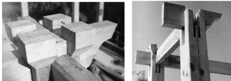
Fig. 1. The construction process by assembling prefabricated components.
