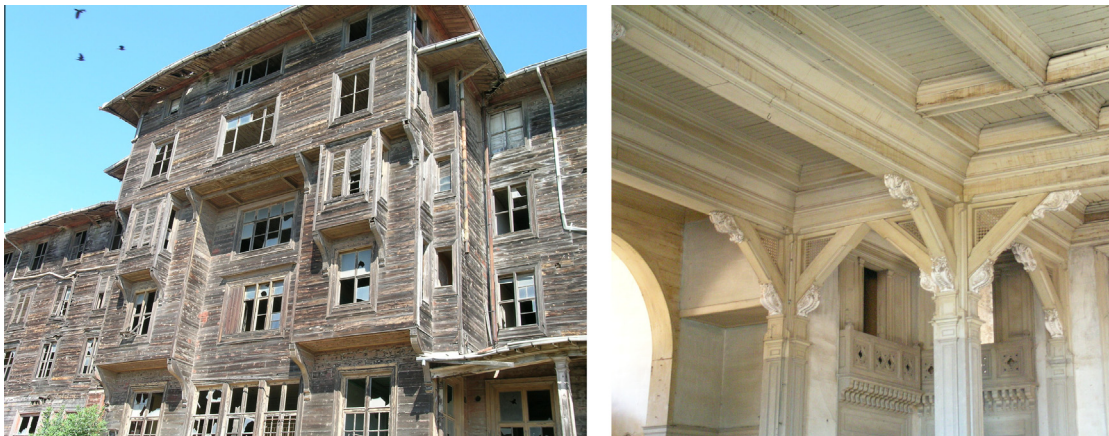
Fig. 1. The Prinkipo palace (left, the façade; right, interior view).
