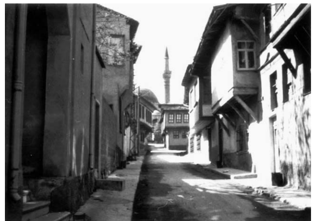
Fig. 2. Buildings with traditional architectural characteristics.
