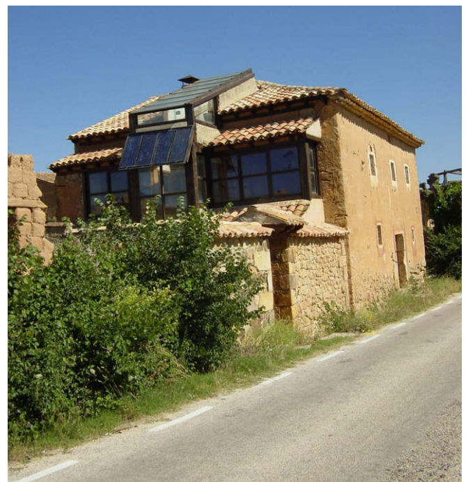
Fig. 2. Southern facade of stone house showing the glazing surface and the solar panels.
