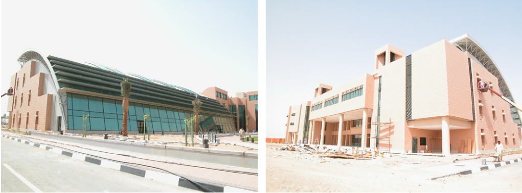
Fig. 1. Pictures of the case study building; north façade (left), south façade (right).
