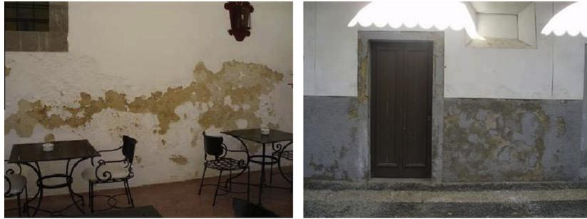
Fig. 1. Decay of renders on the walls due to the presence of soluble salts.
