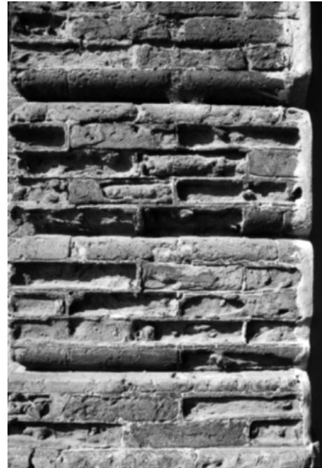
Fig. 3. Decay of the bricks in the portal of the clock tower.
