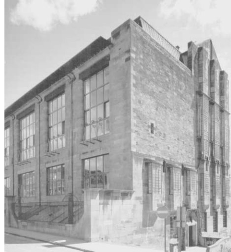
Fig. 1. A view of the GSA building showing the large windows of the north facing studios.
