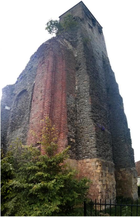
**Fig. 1.** Tower ruin in Dudzele as seen from the northwest. The lower façade is mainly built with buff-coloured limestone, the upper masonry with fieldstone and parts in brick.
