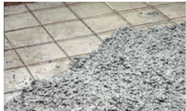
Fig. 4 Topping above hollow cores strips.
