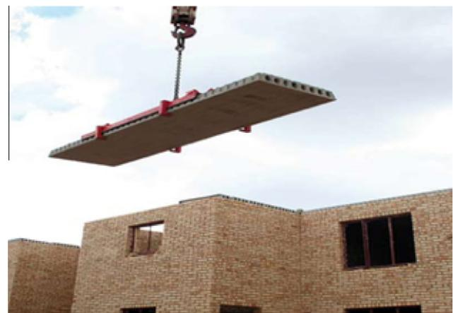
Fig. 3 Installing hollow core strip slabs.
