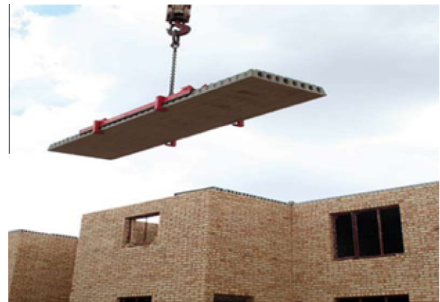
Fig. 3 Installing hollow core strip slabs.
