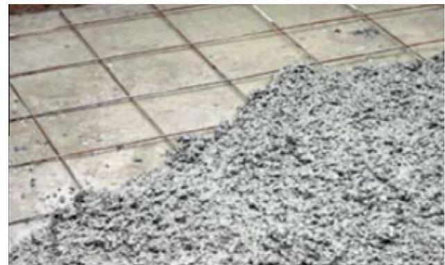
Fig. 4 Topping above hollow cores strips.
