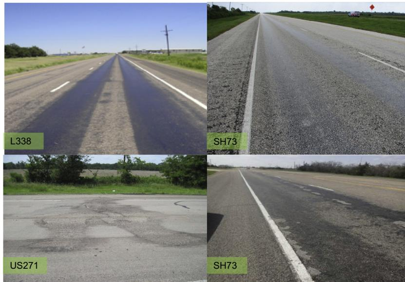
Fig. 1. Candidate pavements for Very Thin Overlays (VTO) with bleeding and raveling surfaces.
