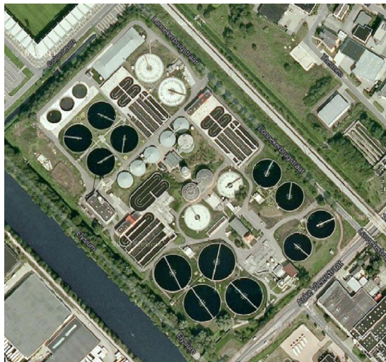
Fig. 1. A bird's eye view picture of the sewage treatment facility in Enschede, the Netherlands. The picture is retrieved using Google Maps.
