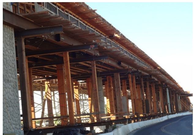
Fig. 4. Bridge falsework (Del Paso Park Overhead, Sacramento).
