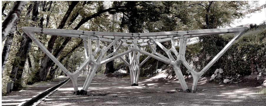
Fig. 1. A photograph of the built structure in Sa'dabad Complex, Tehran, Iran.
