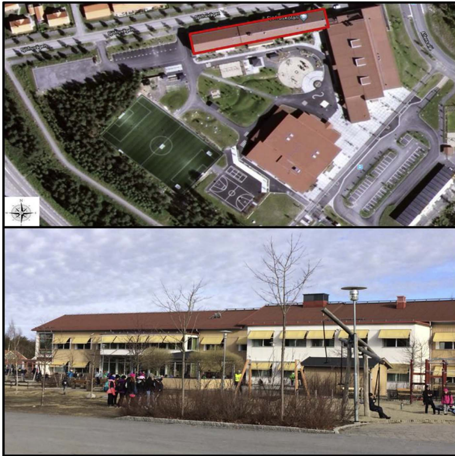
Fig. 1. Diagrammatic plan and photo of the Primary school (Sjöfruskolan) in Umeå, Sweden.
