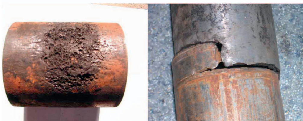
(b) Tubing and casing corrosion fracture pattern
