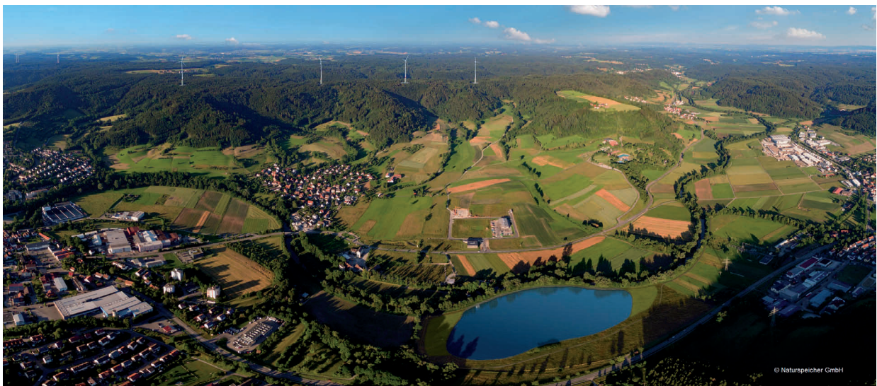
This shows how the landscape around the town of Gaildorf will look at the end of 2018 when the Naturstromspeicher is in full operation.
