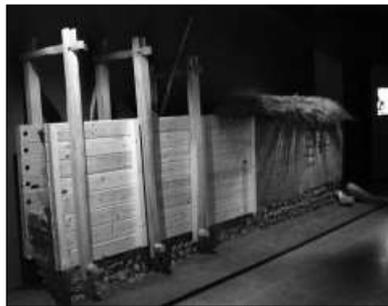
Figure 1: Rammed earth construction [4]
