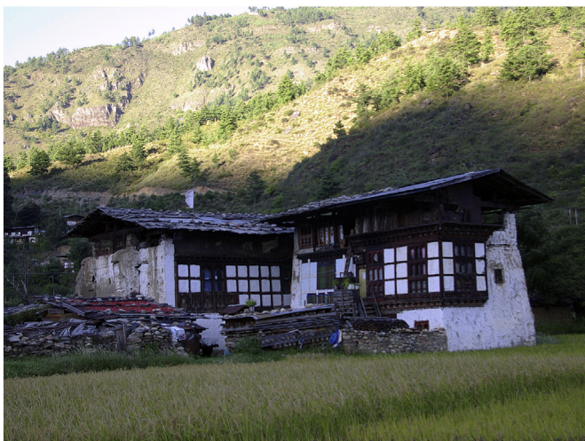
Fig. 1. Traditional farmhouse constructed with rammed earth in the Paro valley in the western part of Bhutan, however with some modifications to the traditional façade structure and roofing.
