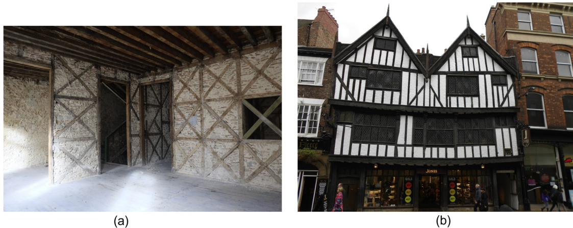
Fig. 1. (a) Frontal walls in (a) Pombalino building (© Stellacci) and (b) timber-framed house in York, UK, XVI century (© Poletti).
