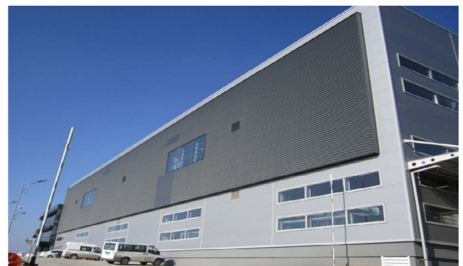
Fig. 1. Building-integrated solar heating systems in factory complex.
