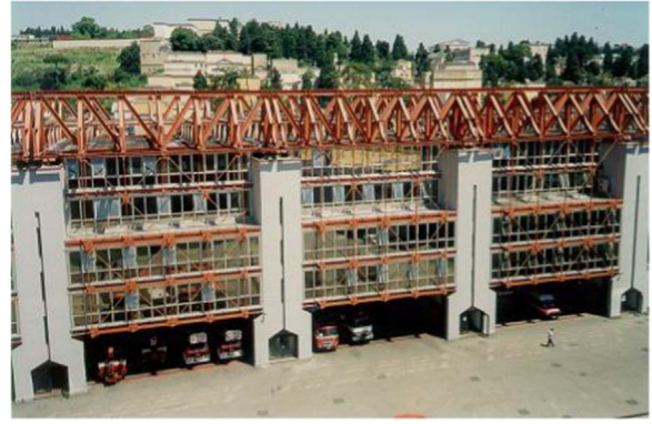
Fig. 4. The first seismically isolated fire-command building in Naples (courtesy F.M. Mazzolani).
