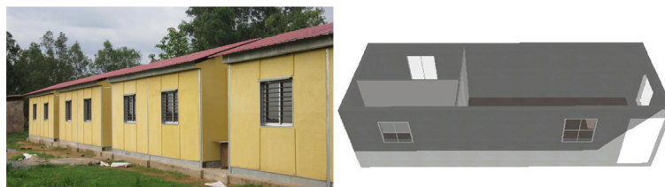
Fig 1. A typical commercially available low-cost modular house in India and its CAD model. [1]
