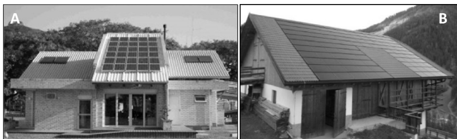
Fig. 1. (A) Photograph of rooftop BAPV realized in Florianopolis, Brazil (Santos and Rütther, 2012) and (B) Photograph of rooftop BIPV realized in Badia, Italy (GSE, 2012).
