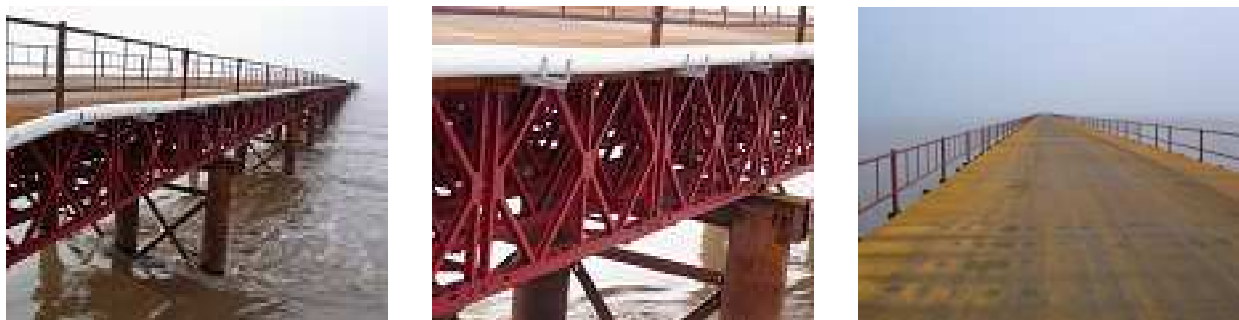
Figure 1. Temporary bridge for constructing Hangzhou bay bridge
