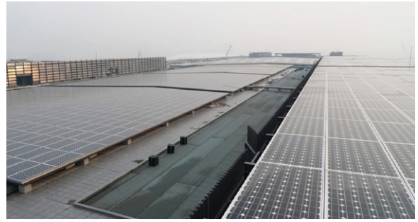
Fig. 2. An example of BAPV in which photovoltaic arrays are attached to the rooftop.
