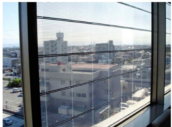
Fig. 3. Effect of amorphous silicon thin-film photovoltaic modules.
