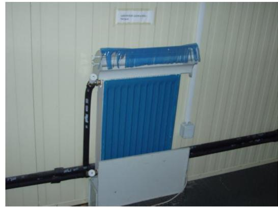
Photo 2. View of radiator-ventilator system.
