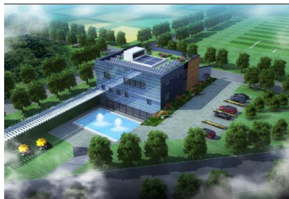
Fig. 1. the appearance of the building.
