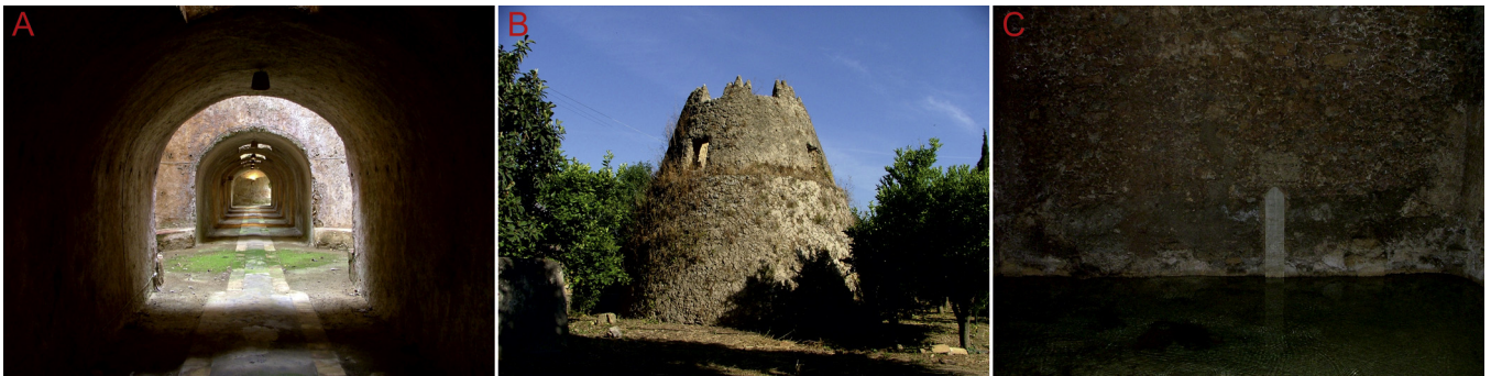
Fig. 1. Ambleri Sirocco room's three main elements. A. Major gallery, mid-internal view. B. Wind tower (medieval water well), external view. C. Large Fountain – the marble plate is a double-measurement device: it indicates the level of the water in the basin along with the water flow rate expressed in the abolished Sicilian unit zappa ( 63 \text{ m}^3/\text{h} ).
