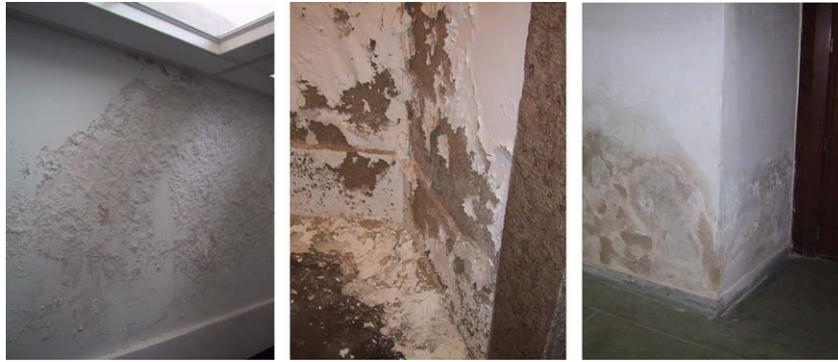
Fig. 1. Different types of surface damage due to salt crystallization: efflorescence (left), physical damage to materials (centre) and dampness (right).
